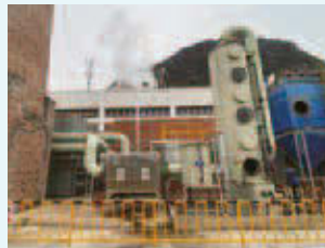
Project site: Linzi, Shandong
